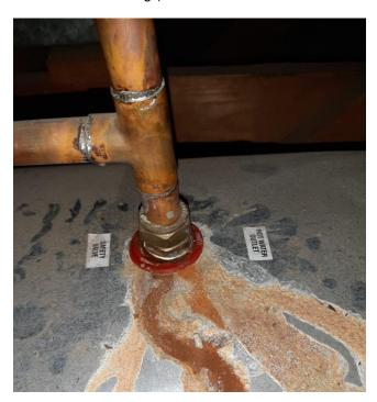
3. TP Safety Valve (Close Up to see color coding for KPA rating and from a distance to show discharge pipe)
