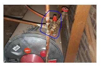
5. Isolation Valve / Stop Valve (This may also be outside not necessarily at geyser depends on Installation)
