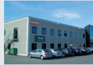
Franke KS Denmark Tilst/Denmark
