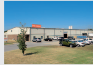
Franke Beverage Systems Inc. La Vergne, TN/USA
