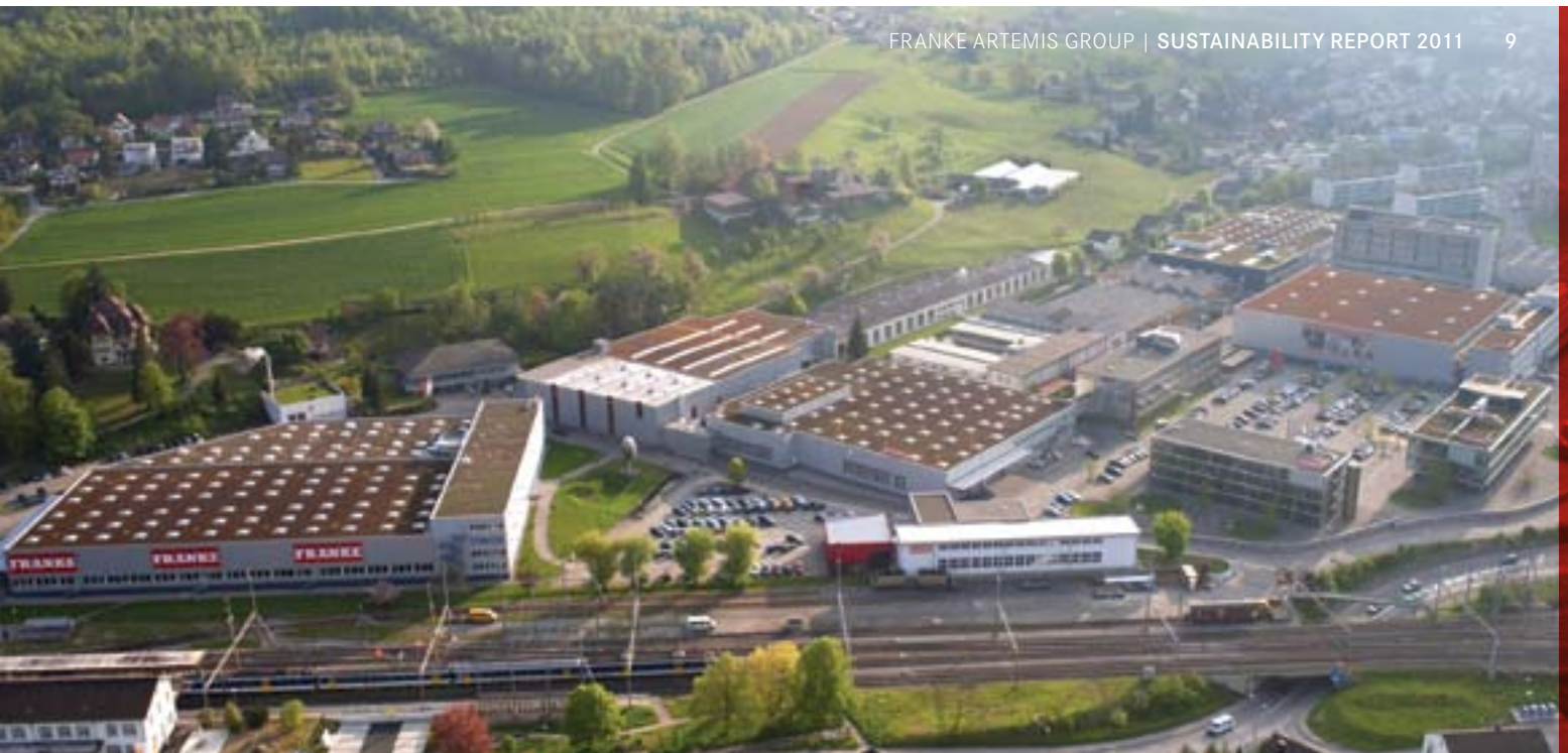
Aerial view of Franke's headquarters and industrial plant in Aarburg, Switzerland.
